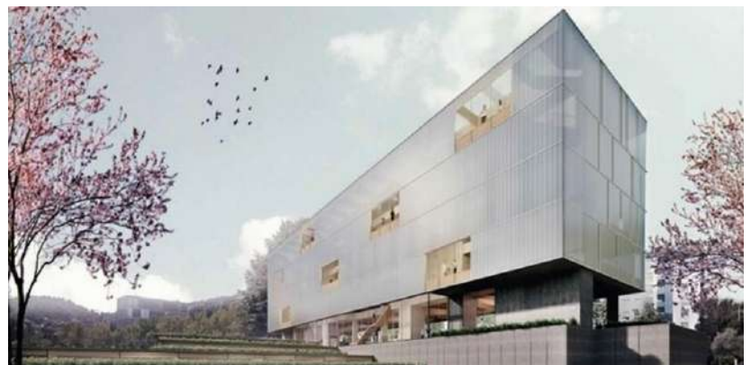
Project for the new headquarters of the School of Aeronautical and Space Engineering on the Ourense campus.
